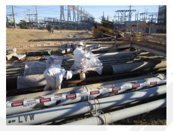
Once all the pipe coverings were removed, windows/drains on the pipes were opened with a non-sparking rivet buster tool to remove the contents and prevent spillage during the piping demolition. The contents were removed utilizing a vacuum truck when possible and transported to the tanks through existing access openings. The demolished pipes were transferred to the tanks for further processing.
